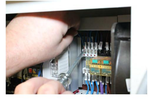
4. 4351 wire goes to A2 - of the relay previously installed.
