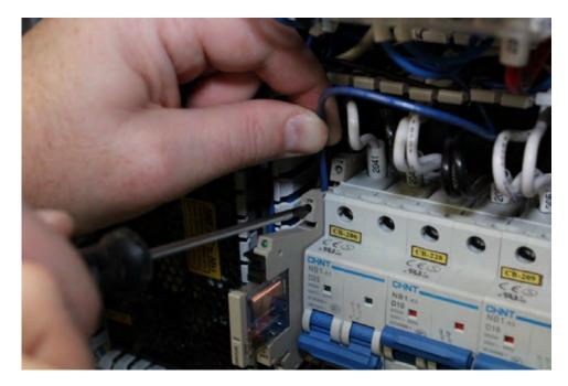
5. Remove white rubber from stripped wire assembly.
