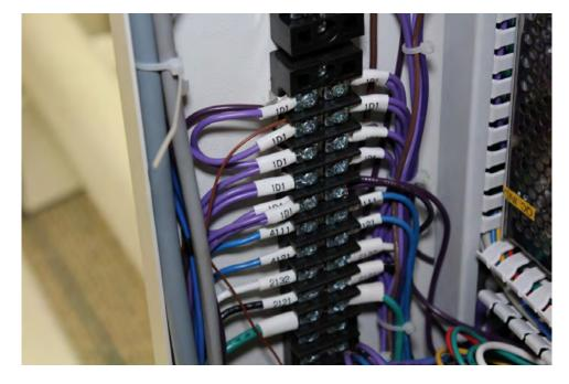
8. The greem wire of the 8 conductor cable goes to ground.
